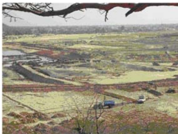
Fig. 17. Sedimentation tanks in the lake bed.
